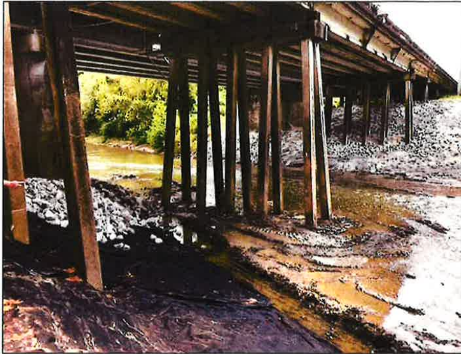
Bridge Piers after Rip Rap and Grouting to prevent erosion in the future
